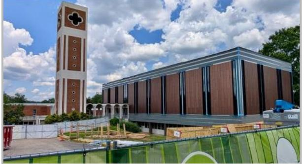
Progress has been made in attaching all the copper panels. The white panels will arrive shortly and will be attached to the top and bottom of the sanctuary building. The "Y-side" stairs will be removed, and work will commence to replace them.
